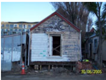
Relocation Preparation - 30 June 2005
