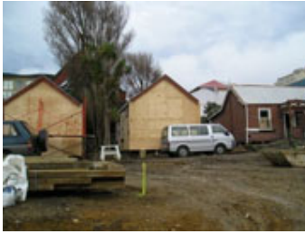
Relocation Preparation - 8 July 2005
