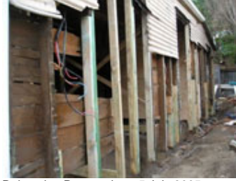
Relocation Preparation - 5 July 2005
