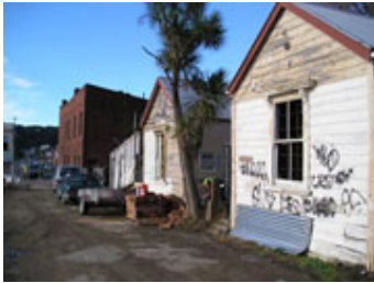
HPT Investigations - 24 June 2005
