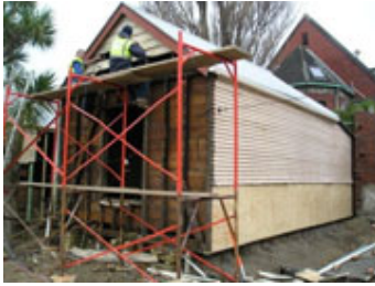
Relocation Preparation - 5 July 2005
