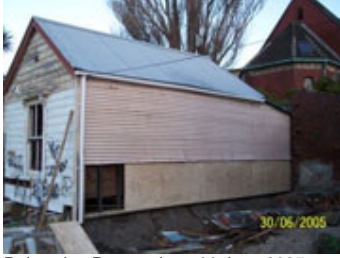
Relocation Preparation - 30 June 2005
