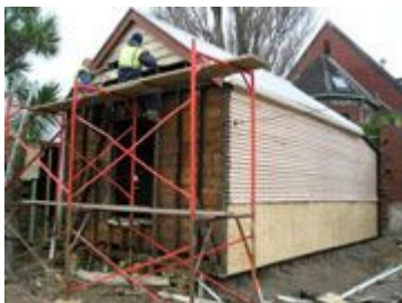
Relocation Preparation - 5 July 2005
