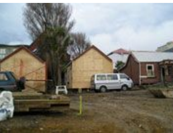
Relocation Preparation - 8 July 2005
