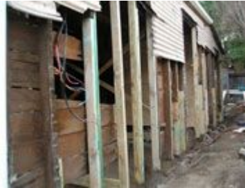
Relocation Preparation - 5 July 2005
