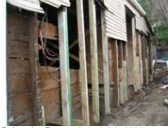
Relocation Preparation - 5 July 2005
