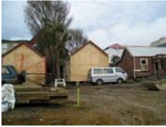
Relocation Preparation - 8 July 2005
