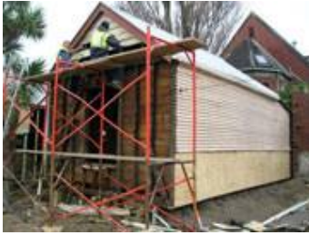
Relocation Preparation - 5 July 2005
